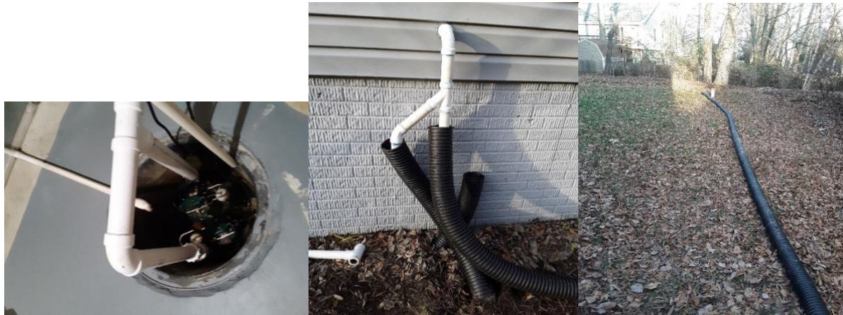
Sump in the basement
